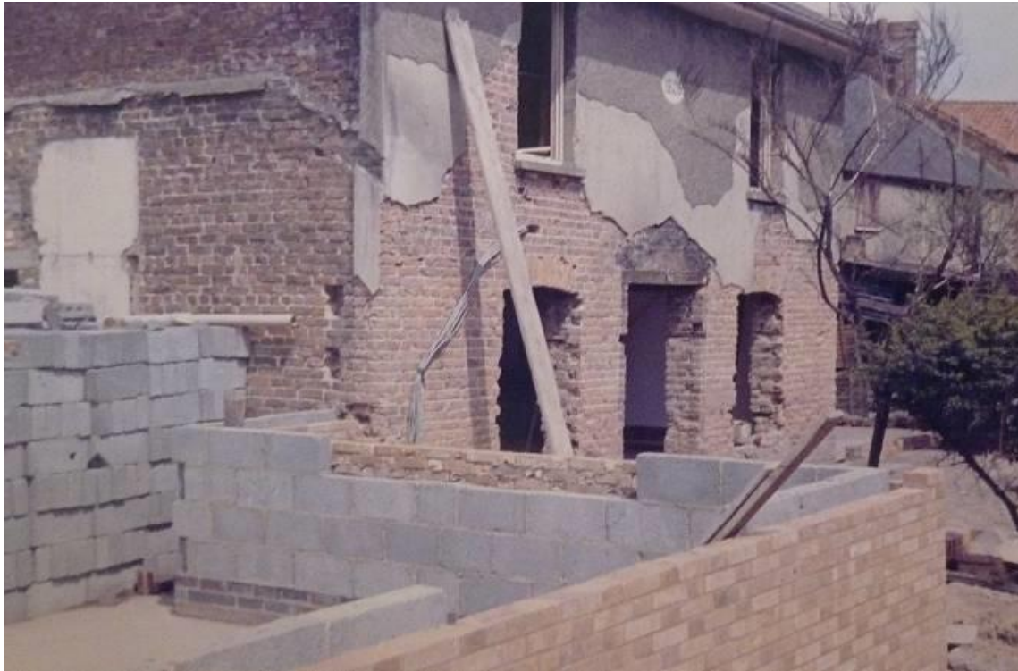
Fig.2 The meeting house during the 1966 refurbishment (Meeting House collection)
